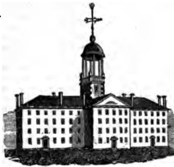
Original University Building.
